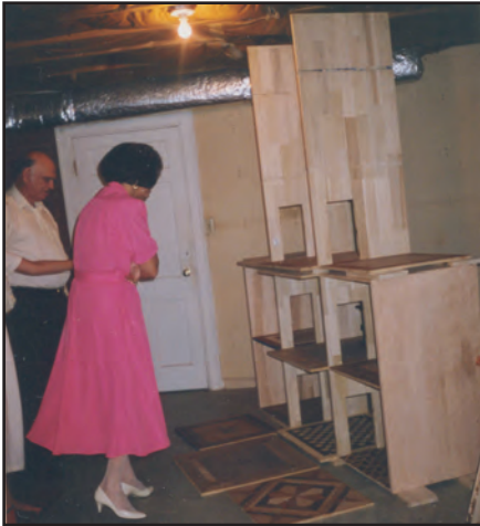
Bird's eye maple house under construction.
